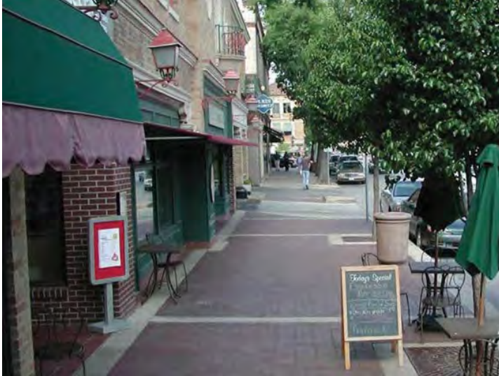
Driveway across sidewalk identified by material change.
