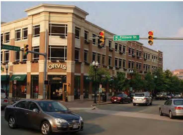
Ground level retail use wrap and compatible façade on upper stories of parking structure.
