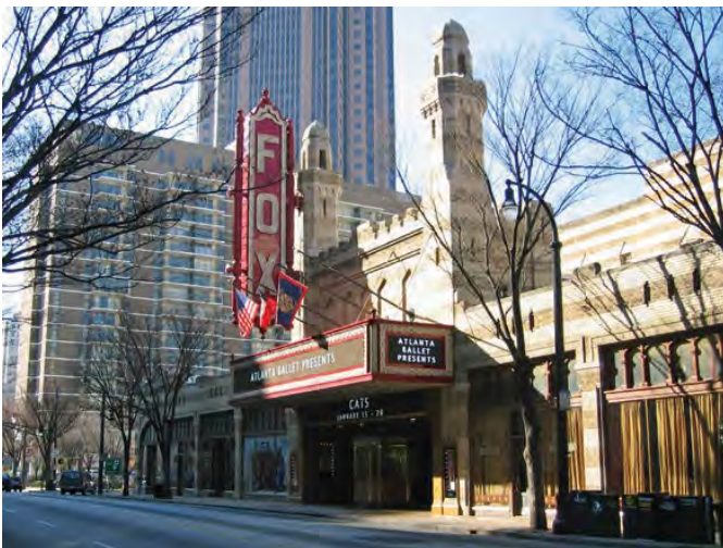
Primary building entry oriented towards street.
