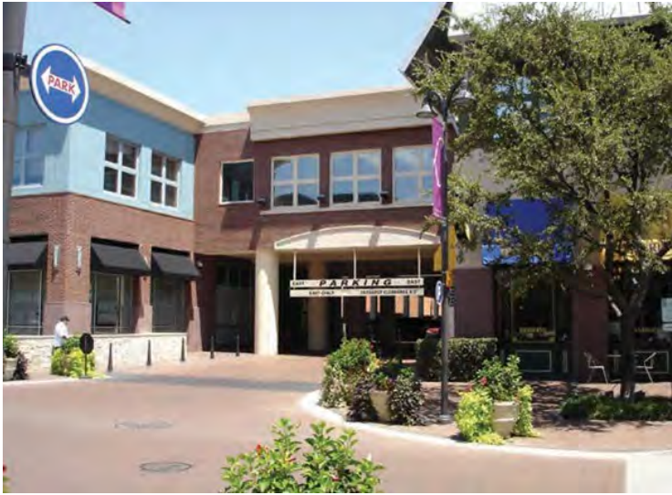
Opening of parking structures should be vertically and horizontally aligned with surrounding structures.
