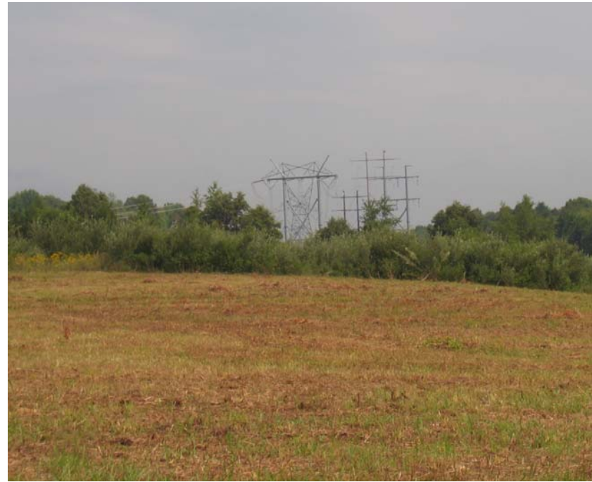
Both types of high voltage power lines now existing on the battlefield are shown above. Both types average approximately 100 feet in height.
