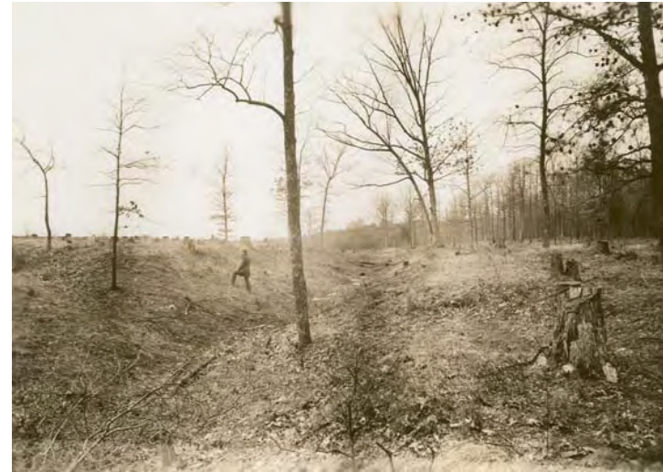
View of unfinished railroad bed looking southwest, 1940. Note the clear terrain just sixty-eight years ago. Courtesy Manassas National Battlefield
