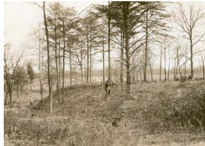
View of unfinished railroad bed looking east, 1940. Courtesy Manassas National Battlefield
