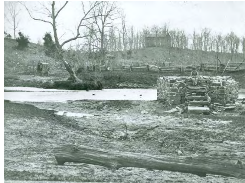
View southwest from Sudley Ford toward Sudley Church (in trees at right center distance), 1862. The viewshed point is on the distant ridge just to the left of the church. Today, this view is obstructed by trees. Courtesy Library of Congress
