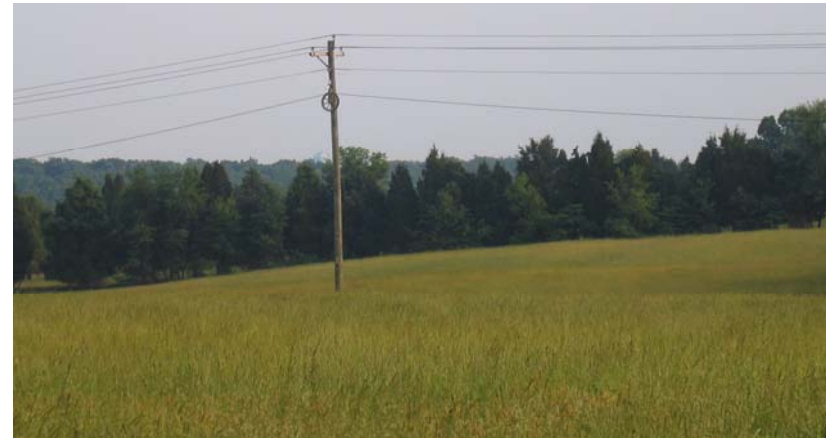
This type of conventional utility pole and overhead wiring exist throughout the battlefield area along roadways.
