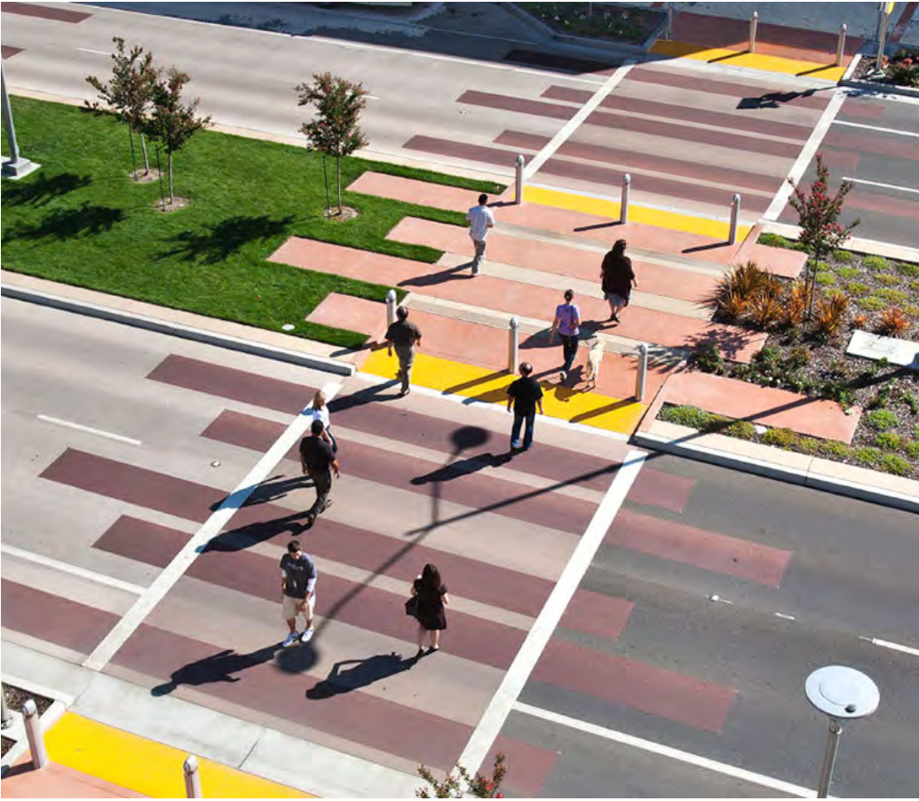
Improve east-west pedestrian crossings along Sudley Road, utilizing enhanced medians as a pedestrian refuge.
